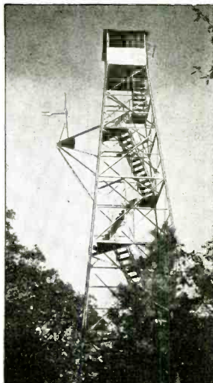
District Ranger Station, Waterton Lake, Glacier Nat'l Pk., Mont. Note windcharger on extension at left.
