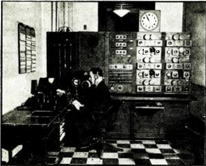
The Board at R.C.A.C., 66 Broad St., N. Y. C., through which all international programs are cleared to the networks.
